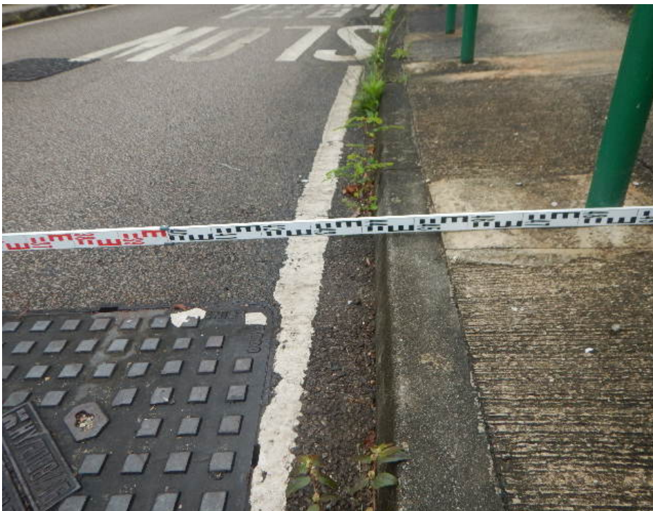
Photo No. A2
