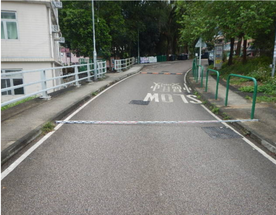
Photo No. A1
